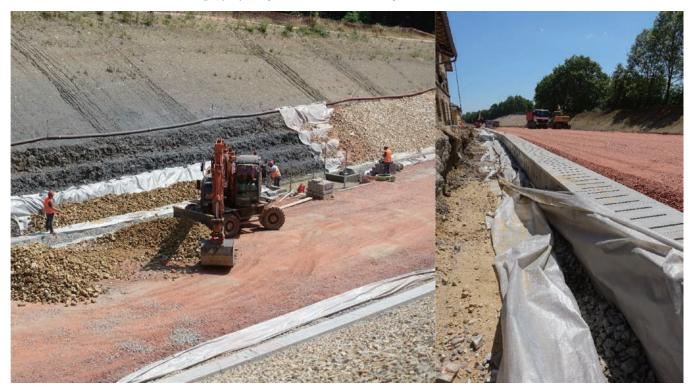
**Project :** Doubling of the railway line between Luxembourg and Sandweiler-Contern. The preferred choice of geotextile was **Typar**® SF for separation, stabilization and drainage.
